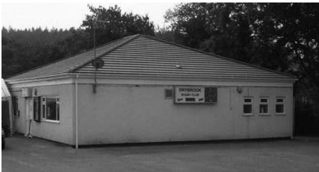
The completed project
