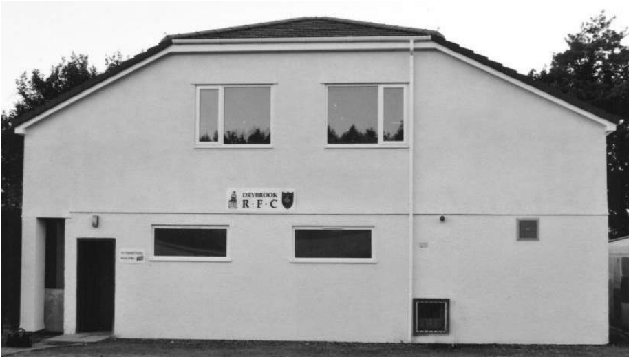
The completed Changing rooms upgrade with new players gymnasium above.
